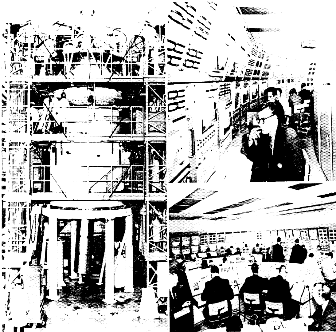
P-276 Checkout at Downey; technicians check cabling to command and service modules (left), while others monitor responses to stimuli on battery of computerized display equipment
